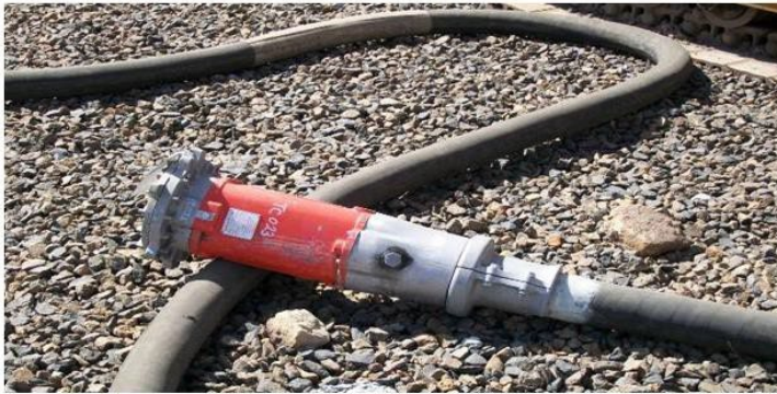
Photograph 8: Plug kept off the ground
