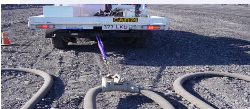
Figure 14: Light vehicle with cable puller
