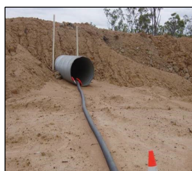
Figure 24 Permanent Cable Crossing – Pipe
