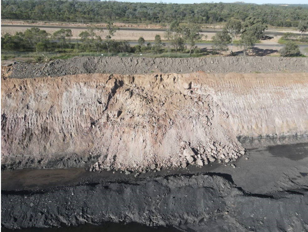
Figure 2-5: Dyno Pit – Highwall Slump – Aerial Photo
