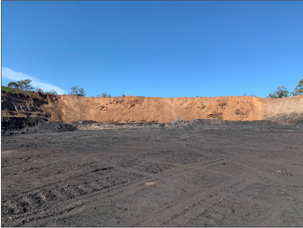
Figure 2-7: Dyno Pit – Topsoil Backfill
