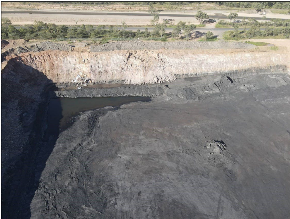
Figure 2-6: Dyno Pit – Highwall Slump – Aerial Photo
